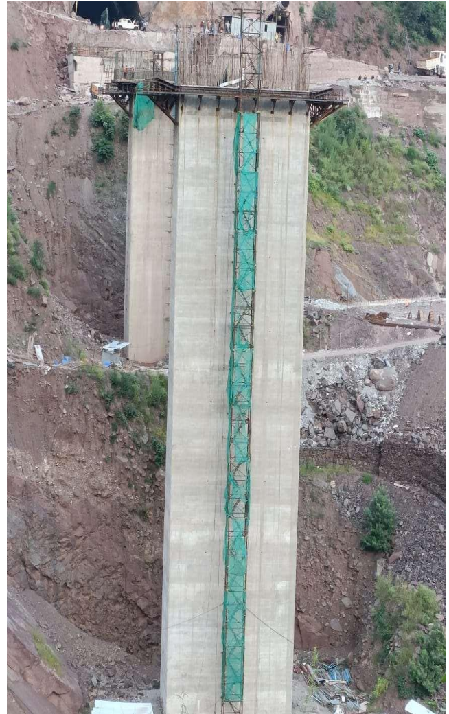
Fig: Pier Construction
