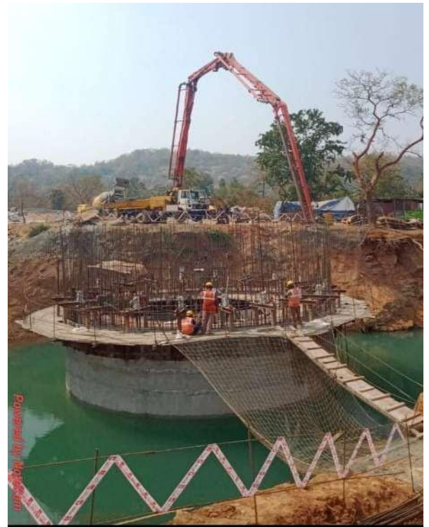
Fig: Intake Well at Rengali Dam
