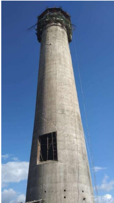
Fig: 50mtr. High RCC Chimney at Jai Balaji
